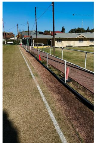
This work has been undertaken largely by one member. The purpose of the work is to address the issue of balls becoming airborne when crossing the boundary of lawn 3 and to remove the deteriorating wood sleepers, while hopefully allowing an unimpeded shot from the western boundary.
